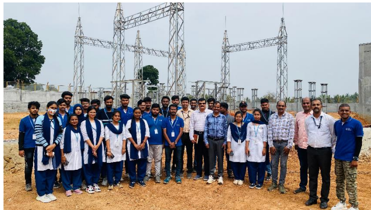
Pic: Substation site visit at Mara Gowdan Halli 66/11kV Substation in KR Nagar Taluk, Mysuru
