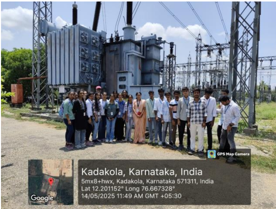
Pic: 4 th semester students at 220kV kadakola Substation, Mysuru
